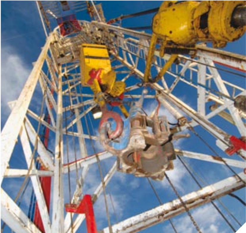
Top left: Welding at the main compression plant at Berwyndale South. Top right: Gas and water gathering pipelines are buried underground, leaving little evidence of the gas production process. Main picture: View to top of Ensign rig #34.
